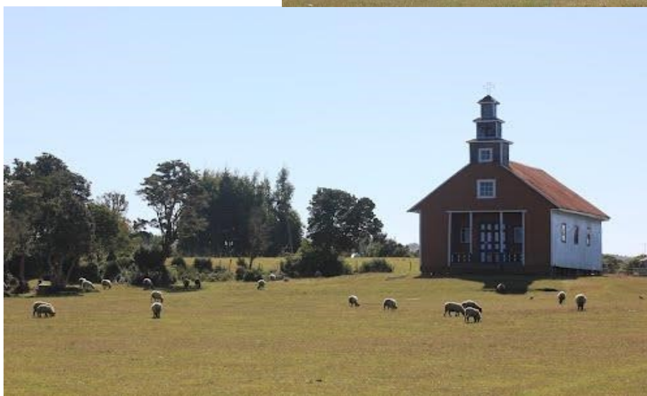
Chiloe wooden church near Cailin
